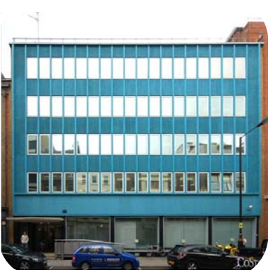
68 Newman Street, London W1 Lease Disposal for ABTA
